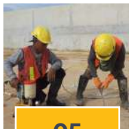
PRESSURE GROUTING
